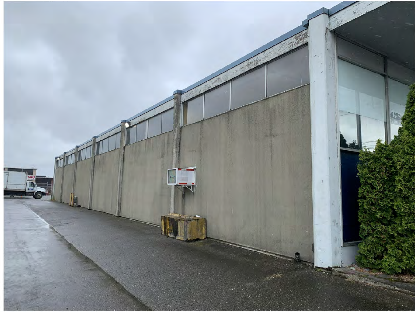
2 PHOTO - EXTERIOR ELEVATION E NTS
