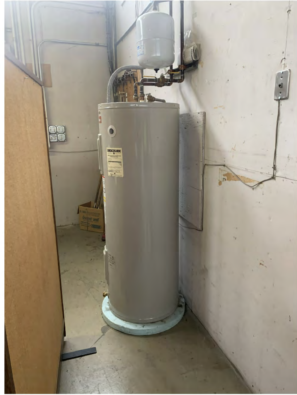
5 PHOTO - STOR AREA INTERIOR NTS
