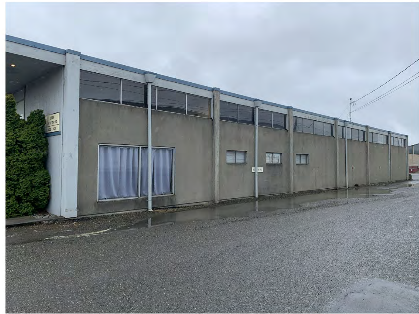
4 PHOTO - EXTERIOR ELEVATION W NTS
