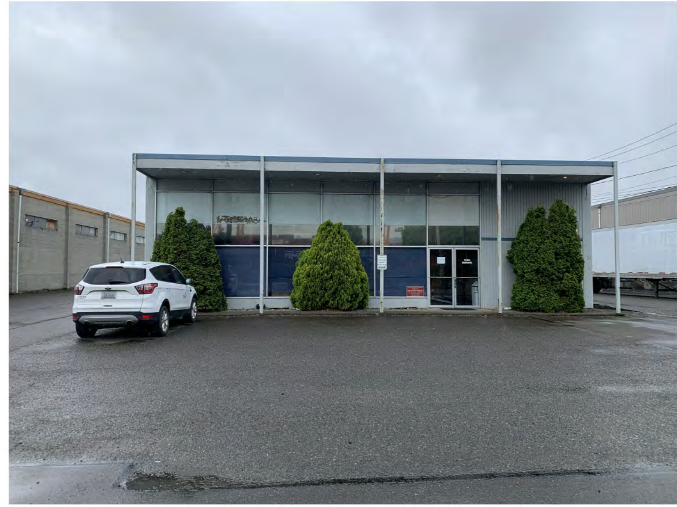
1 PHOTO - EXTERIOR ELEVATION N NTS
